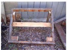
Take the two 26in sections and two 34 1/2in sections and nail screw them into a square shape
