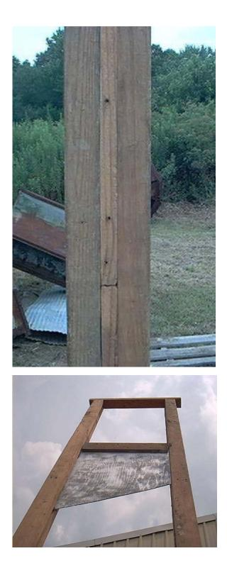
The guillotine blade tracks are made from 2 2X4s nailed face to face with a strip of 1X2 lumber at on edge between them. This gives you the 3/4" gap for the blade to run up and down in.
