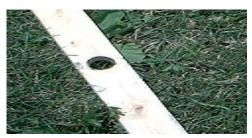
This is the hole through the platform for the shaft of the motor and the crank. The hole was drilled with a 5/8" spade bit. I drilled about 1/2 way through the 1X2 with the bit and then flipped it over and drilled the rest of the way through to prevent splintering.
