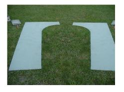
The remaining two pieces of plywood from cutting out the doors would be the entrance archway. They were painted with an oil based paint. (Remember, they need to be water resistant, this is all going to be outside.) Color = grey
