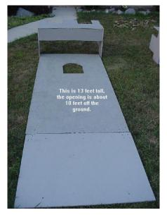
At this point the tower was only 8 feet tall, I needed more height! I cut out two 3' x 4' sections from the sixth piece of plywood. This gave it a total height of 11'. Add another 2' for the turret and the towers total height is now a whopping 13' tall!
