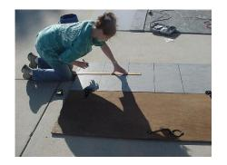
Using a T-Square and a pencil, create a brick stone pattern (Each brick was 2 ft wide, and 1 foot high.) After drawing the pattern in pencil, we went back over the lines (still using the T-Square) with a permanent black marker. (We decided to use that instead of a paint brush because the paint brush method tended to **NOT** be as 'neat and clean'.
