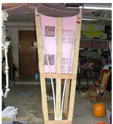
I then ran pvc pipe from the ground up the back to the top corners of the chair for hooking up a fog machine to shoot fog out.
