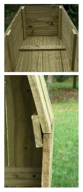
The upper sidewalls were screwed to the vertical ribs and the sidewall support pieces attached to the bottom.
