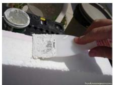
Because I'm a psychotic OCD perfectionist type, I like to fill in all the gaps where the two foams are glued together. I just use joint compound and a plastic putty knife to do this. It's not a necessary step, but I like to do it anyway. I sand it smooth when it's dry.
