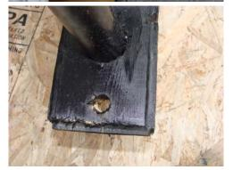
This is the hole drilled in the bottom cross member that the fence lag inserts into.
