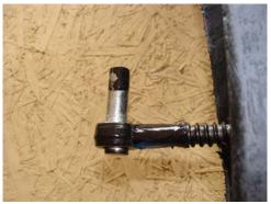
Here is the fence gate lag used as a hinge.
