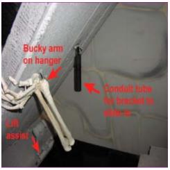
This shows the attached piece of metal conduit on the top of the crypt.
