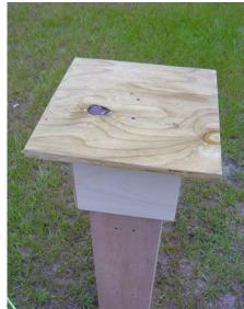
Wood glue and finish nails hold the block in place while the glue sets. This joint will be part of the fence post's structural integrity, so a good fit here is important.
