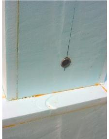
The center of the top hole is located on the crosshair drawn in the last step.
