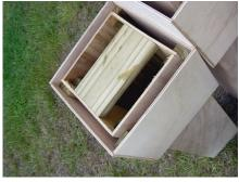
A 1X4 support block is added to the bottom of each post, inside the center column.
