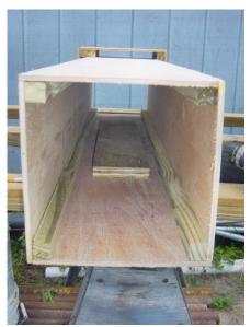
3/4" plywood backing boards are added to the inside faces of opposing walls.
