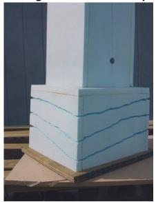
There is something about the look of field stone ... so I decided to mimic that effect on the bases of these fence posts (hence the extra foam thickness in this area.) Beginning with a dremel tool and a thin tapered diamond burr bit, horizontal lines were carved all the way around the base - generally three lines, but occasionally four.
