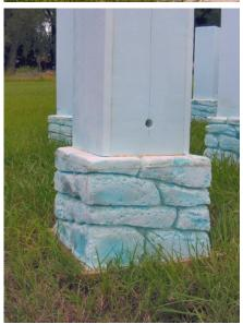
After carving all of the rough lines, I used a sand blaster to break all of the hard corners and begin shaping some of the stones. Depending on how you plan to fine finish this area, you may not want to remove too much material ...just enough for a good start in defining the general shape.
