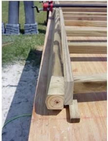
The original jig is disassembled after the last center section is built. Once the glue dries, each section will receive upper and lower 2X4 pieces. The center panel sections rest on (loose) 1/2" thick strips of wood, creating the proper reveal (of equal size) on each side of the fence panel section.
