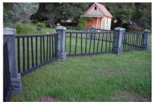
Easy fix with this system - lift the panel out of the sockets, thread the sockets into the post, tighten the nut, and reinstall the panel. The gap is adjustable per intersection!
