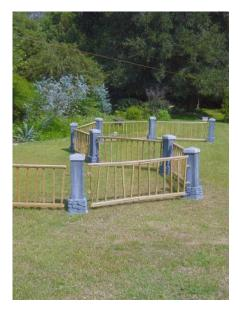
The mounting hardware used with this project allows for varied angles between the posts and panels. This creates a unique effect, as opposed to perfectly straight lines.
