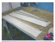
Four identical pieces of 1/4" luan receive nailer blocks. These are glued and nailed in place along one side of each plywood wall. Whether you start with the left or right side doesn't matter as long as all pieces are the same for each column.
