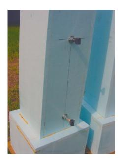
All that's left to do is hold the back nuts/connecting rod assembly in place while the threaded rods are started in from the outside. Once positioned properly, the outside nuts can be tightened fully.
