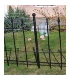
Spray post and ball black to match your fence panels (you can save time and money by constructing the posts with 2" black PVC pipe saving the trouble of having to paint the posts)
