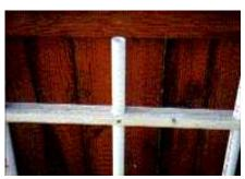
Now you will need to fasten the pipe and lumber in place. The easiest method is to pound a finishing nail though the wood into the pipe. A sturdier method is to drill a hole though the wood and pipe, and use a wood screw to fasten the pipe in place as shown on the right below.
