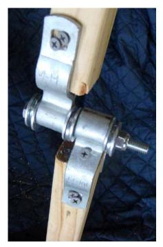
I found that my hinges needed another set screw to keep them from rotating out of square... So I drilled a new hole, and zipped in another deck screw
