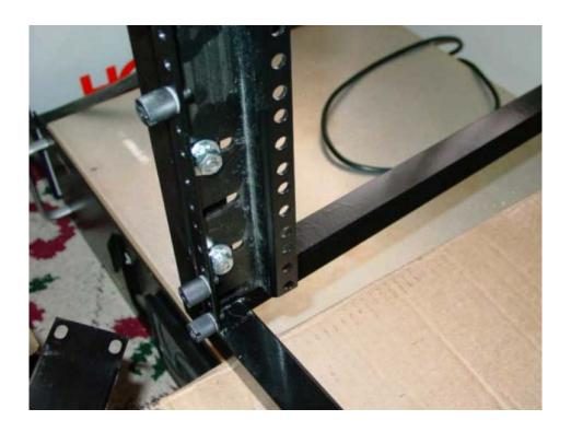
Each rail is mounted with four 1/4-20 bolts, flat washers, lock washers, and nuts. An additional flat washer is placed between the rack rail and the frame itself in order to make sure the space between the rails is proper to produce the required horizontal mounting-hole spacing of 18 1/4". The rack rails are then checked to ensure they're level vertically as well as the right distance horizontally, and then hardware if tightened down to complete the installation.
