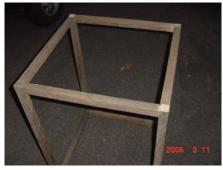
The fan must be enclosed on all sides except the intake and exhaust in order to channel the air properly. In the pics below you can see how we mounted the fan, and began to enclose it with wood framing to channel the air.
