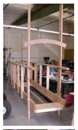
The final version of the bridge was a little different than these pictures show. The walking surface of the bridge was moved up to the middle of the side 2x10's which allowed us to run 2x4 bracing underneath to strengthen the hand rails. The final version is a **very** solid structure.
