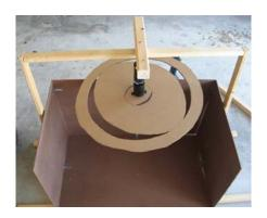
**Description:** Now for the pulsating part. I want the meteorite to be enclosed in a metal box with a window. So I got some 4x8 "hard board" from Home Depot and had them cut it to size. I used brackets to bolt the sides together and constructed a support over the top of the box (which will remain open).
