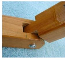
The legs consist of wooden 2x2's (approximate dimensions below). The leg joints are just simple tongue and groove cuts joined by a #10 screws, washers and nuts.
