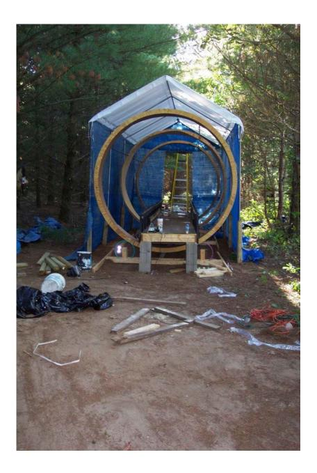
Now that the tunnel is assembled, we needed a way to cover it. Rain water collecting on the tunnel itself could lead to major problems, so if you have this outside, you really need a cover. This is a 1 car portable carport that we picked up from Menards for a hundred bucks. It wasn't quite tall enough, so we buried some 8' posts, and mounted the garage to that. Large pieces of blue tarp make up and front and sides of the tunnel.
