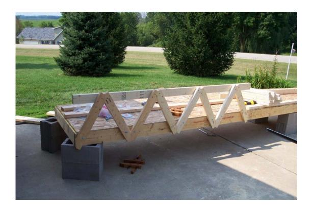
Enter the removable trussing. All of this is built with 2x4's and bolted to the bridge. Each side is made up of 3 8' sections of trussing.
