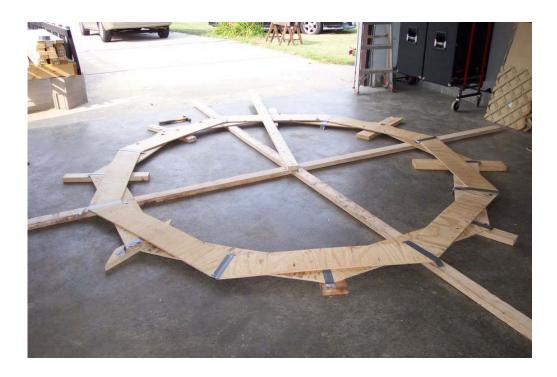
Here, we have arranged the second layer on top of the first. This needs to be offset, to the break of two borads on one layer will be the middle of a board on the other layer.
