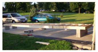
Here is a photo of the side of the bridge. This is both the 12' sections, bolted together in the middle.
