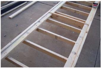
Here is a photo of the first section with the 2x4's in place. Remember that this is upside down.
