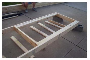
Also, we take two additional 2x4's and run the flat on the underside of the bridge, which will give us something to mount our handrail to.
