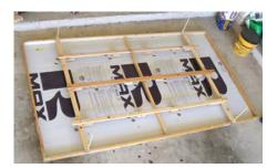
Next, I made the frame that would hold the spikes. It was essentially three crossbars held in place by two connecting boards. I drilled a good size hole in each end of the connecting boards and reinforced the end with a metal bracket. These holes fit over the threaded rods. and acted as guides. I used wood screws to attach 12 wooden blocks on the underside of the spike frame (they were spaced about 1.5 feet apart.
