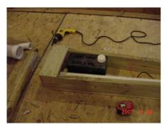
We cut a sheet of plywood to cover the bottom, and cut one of the planks that will cover the top just to hold things together while we sized everything up.
