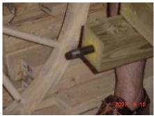
We purchased 12" lengths of 1/2" black pipe and cut them in half (two 6" long pieces). We then drilled a 7/8" hole into each axle to insert the pipe.
