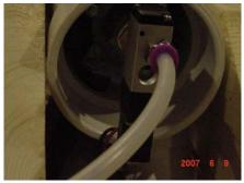
The QEV is connected via a 3/4" x 8" steel black pipe to the holding tanks below. I had to drill a hole on the underside of the 4" PVC barrel" for the black pipe to pass through.
