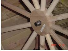
A 1/4" x 4" bolt with nut run through the axle holds it in place.
