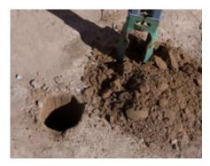
Dig a one foot deep hole large enough in diameter for the base of the mast to fit into. You can use either a shovel or a post hole digger like we did to dig the hole. Slide the base of the mast into the hole and fill with dirt. Tamp the dirt down around the board firmly to make a secure foundation.
