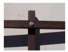
Drill a hole in the center all the way through both boards. Push a bolt all the way through from the top to the back. Put a washer and bolt on and tighten.
