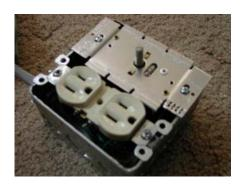
Removing the cover plate, we see a standard two-outlet electrical receptical.
