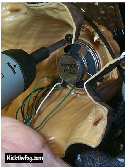
With the panel removed, remove the screws that hold the speaker.
