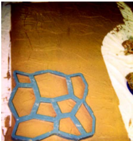
Using the Concrete Form to press the stones into the joint compound
