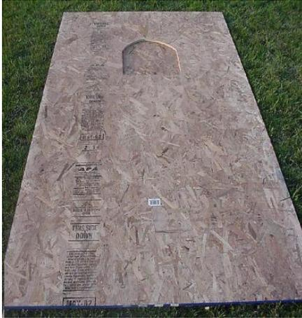
Of course, every castle needs towers, I cut out a small window in the towers using a jigsaw, after I cut out the FIRST window, I placed that piece of plywood on top of the other piece of plywood that would become the other tower. I then traced out the outline. Why did I do it this way ? So that the windows would be identical to each other!
