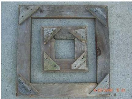
This is the top and bottom part of the frame. I like to screw these together on the top using "L" brackets because I think it holds better (the picture shows 1x4 cut into triangles to hold the boards together but the eventually broke from moving the columns).
