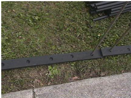
As you can see, we used wood for the bottom and top rails, drilling the holes only halfway through the bottom so when the pvc is inserted, it lays on top of the wood. The top rail's holes are drilled completely
