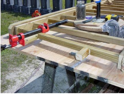
In order to properly align the post hardware and the panel, another jig is used.
