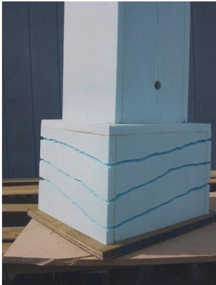
There is something about the look of field stone ... so I decided to mimic that effect on the bases of these fence posts (hence the extra foam thickness in this area.) Beginning with a dremel tool and a thin tapered diamond burr bit, horizontal lines were carved all the way around the base - generally three lines, but occasionally four.
