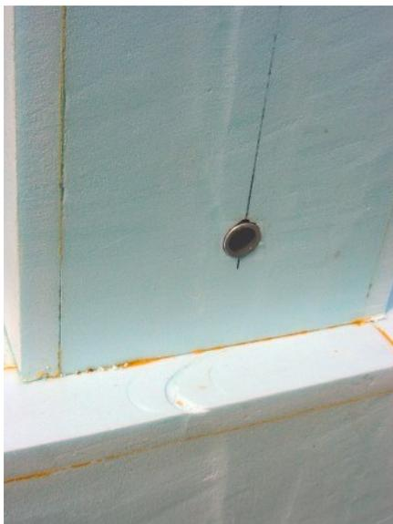
Using this center hole, switch to a smaller drill bit that is slightly over sized for the threaded rod portion of the mounting hardware, but smaller than the pipe spacer's diameter. In this case, a 9/16" hole is perfect.
