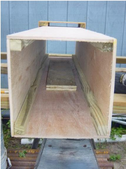
3/4" plywood backing boards are added to the inside faces of opposing walls.
