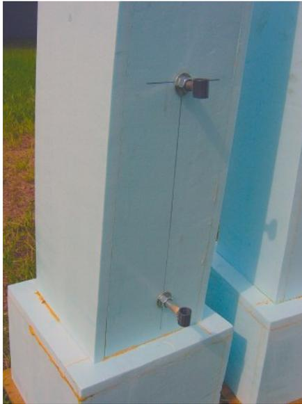
All that's left to do is hold the back nuts/connecting rod assembly in place while the threaded rods are started in from the outside. Once positioned properly, the outside nuts can be tightened fully.
