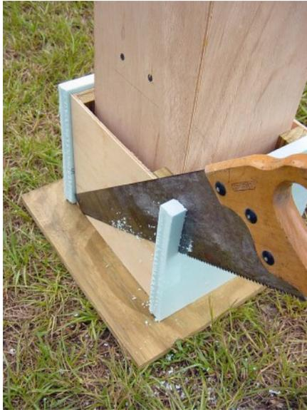
After the polyurethane glue is fully cured, excess sheet foam is easily trimmed with a handsaw. Keeping the saw blade tight to the wood box will produce a tight fitting joint when the remaining sides of the box are covered with sheet foam.
