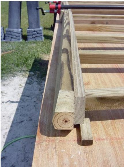
The original jig is disassembled after the last center section is built. Once the glue dries, each section will receive upper and lower 2X4 pieces. The center panel sections rest on (loose) 1/2" thick strips of wood, creating the proper reveal (of equal size) on each side of the fence panel section.
