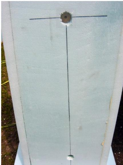
The center of the top hole is located on the crosshair drawn in the last step.
