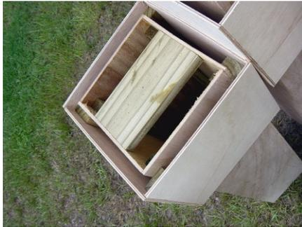
A 1X4 support block is added to the bottom of each post, inside the center column.
