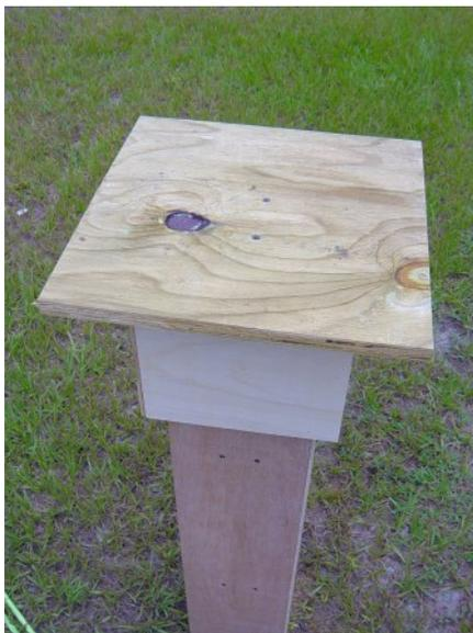
A square plywood base is attached to this support block from the bottom.
