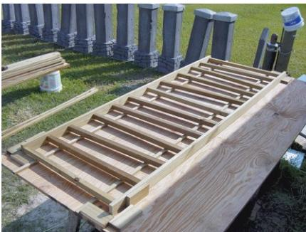
All of the vertical pieces are all cut, glued, and installed between the top and bottom plates.
