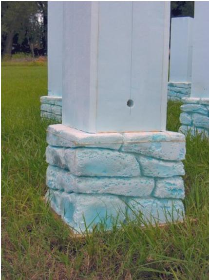
The final stage in the shaping process ... A careful application of heat from the torch softened some of the corners and edges. It also added some inconsistency to the faces of treated stones. To finish off, and in this particular order, a chemical application of acetone causes sporadic pitting anywhere it lands.
