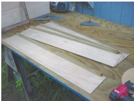
Four identical pieces of 1/4" luan receive nailer blocks. These are glued and nailed in place along one side of each plywood wall. Whether you start with the left or right side doesn't matter as long as all pieces are the same for each column.
