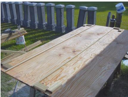
A simple jig is made for panel assembly. For the creation of this jig, scrap pieces of wood are nailed in position marking the maximum location of each corner of the panel sections. Long, thinner strips of wood are nailed in place to hold the vertical pieces at the proper height in relation to the top and bottom plates (ripped during the previous step.)
