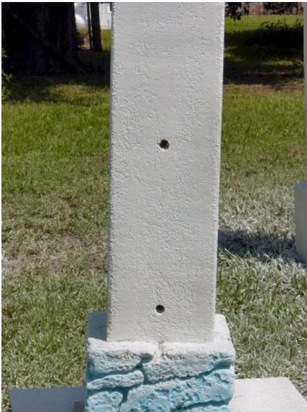
This is not a difficult procedure to master. Shoot a few test pieces on scrap material. Experiment with different joint compound consistencies and air line pressures until you achieve the spray pattern you like.
