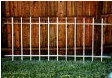
I spaced the 1x2 lumber so it was 5 inches from the top and bottom of the pipe. Experiment with the arrangement and use what looks good to you.
