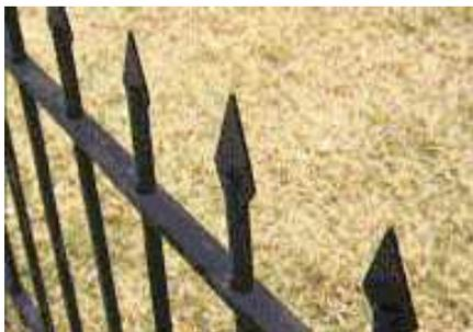
I used 2 sizes of finials, and alternated them across the fence (This only works if you have an odd number of fence bars). I cut slots in the finials to slide them over the ends of the pipe. A quick dab of hot glue held them in place.
