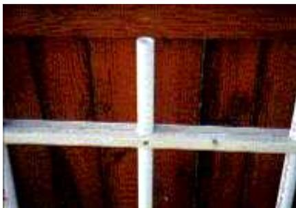
Now you will need to fasten the pipe and lumber in place. The easiest method is to pound a finishing nail through the wood into the pipe. A sturdier method is to drill a hole through the wood and pipe, and use a wood screw to fasten the pipe in place as shown on the right below.
