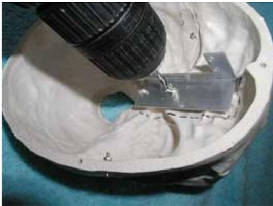
Using the appropriate size drill bit for a #6 screw, drill a hole through the bracket and skull where they were marked.
