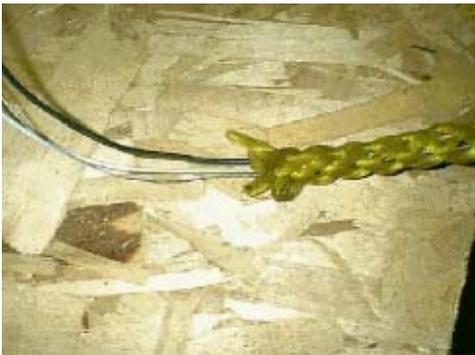
Once your head and hood are in place you will feed the wires through the center of the coreless nylon rope.
