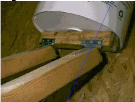
Measuring the bottom of the pail, cut one piece of 2" X 2" lumber to span across the center.
