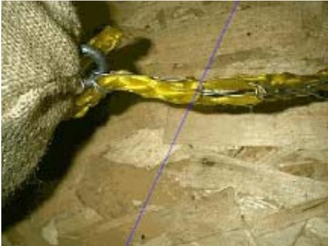
Attach the electric fence wire to the hole in the flat bar on the outside of the hood leaving a few inches sticking out.
