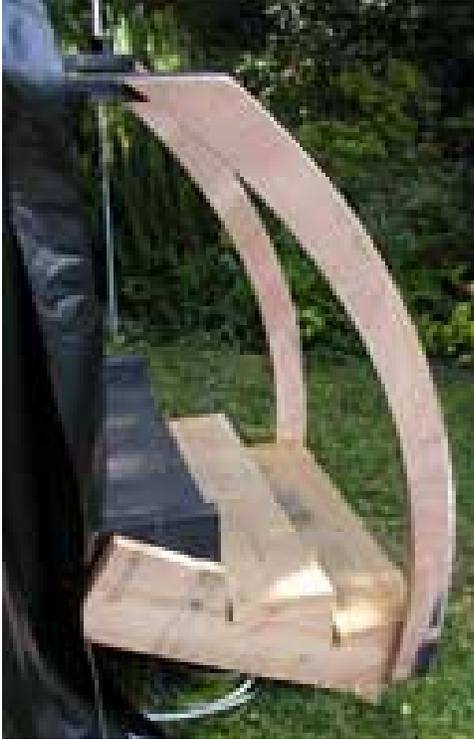
These are the stairs for the bridge. The handrails were made from arcs leftover from our test hoop.
