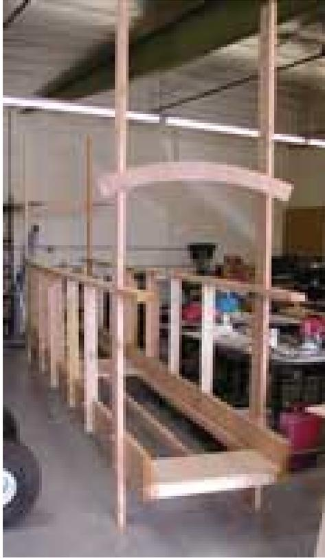
The final version of the bridge was a little different than these pictures show. The walking surface of the bridge was moved up to the middle of the side 2x10's which allowed us to run 2x4 bracing underneath to strengthen the hand rails. The final version is a **very** solid structure.
