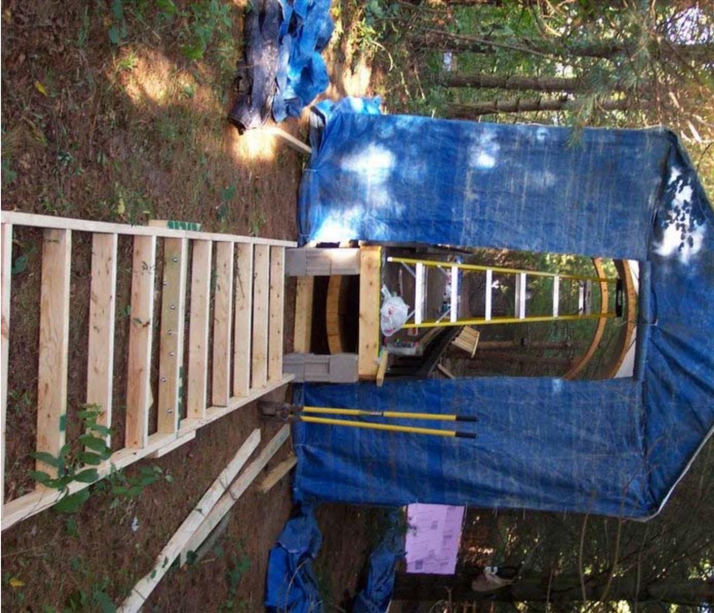
And here is the last photo I have of the construction process. The ramps were built on both sides, and a handrail was installed.
