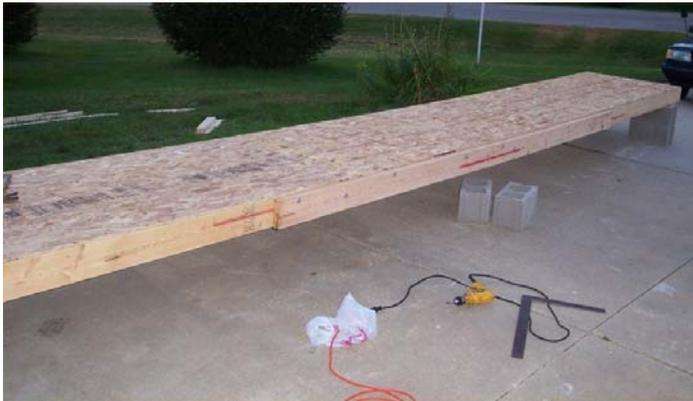
Here it is with the top of the bridge in place. It's made out of 1/2" OSD, but in retrospect, we should have used some metal grating or something. The final effect was still effective, so it worked!
