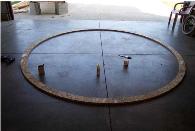
The process of assembling these rings is pretty easy. If you don't have to make these movable, you can just make each ring into two halves, and assemble the halves around the bridge. We needed to move these rings quite a distance in small vehicles, so these come apart into 4 sections.
