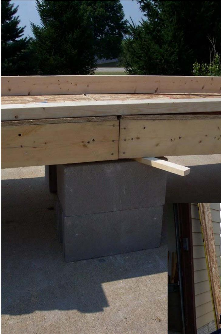
We raised the middle section a little bit while installing the trussing, to give it a bit of a natural arch.
