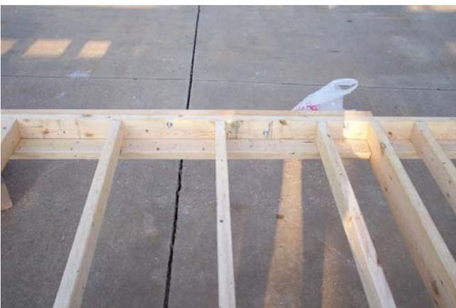
And here you can see the 2x4's that run under the bridge, which gives us something to mount piping to for the handrails.
