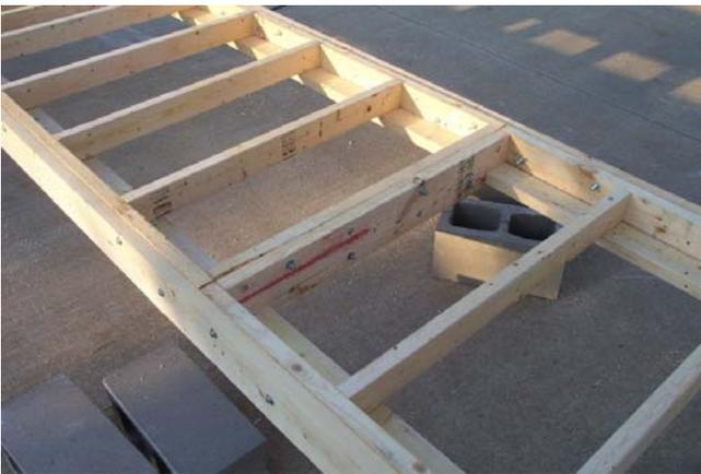
Here is a photo of the connection in the middle. You should notice that we bolted another 2x8" x 12' onto each side of the bridge, centering the plank with the break of the other two sections. This provided quite a bit of support.
