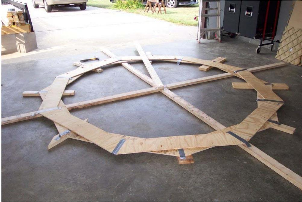
Here, we have arranged the second layer on top of the first. This needs to be offset, so the break of two boards on one layer will be the middle of a board on the other layer.
