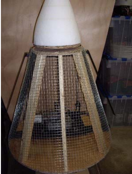
Wire formed over frame and head blank in place.
