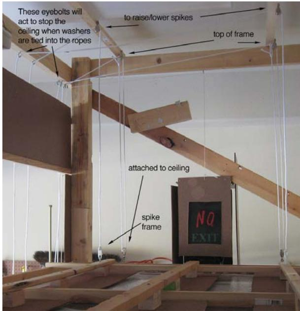
I now had eight ropes to pull (four for the corners of the ceiling and four for the corners of the spike frame). Before I could attached them to anything, I needed to balance the ceiling and frame.
