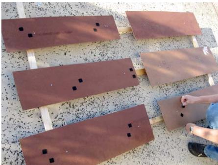
Next, I attached six cut sheets of hardboard to the blocks. I then returned the spike frame to the ceiling and marked where the holes were. I bought a couple of packages of the Velcro sticky pads at the grocery store and placed the adhesive end over the marks. These pads will hold the spikes to the frame, but also allow them to be easily removed.
