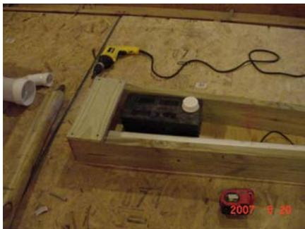
We cut a sheet of plywood to cover the bottom, and cut one of the planks that will cover the top just to hold things together while we sized everything up.
